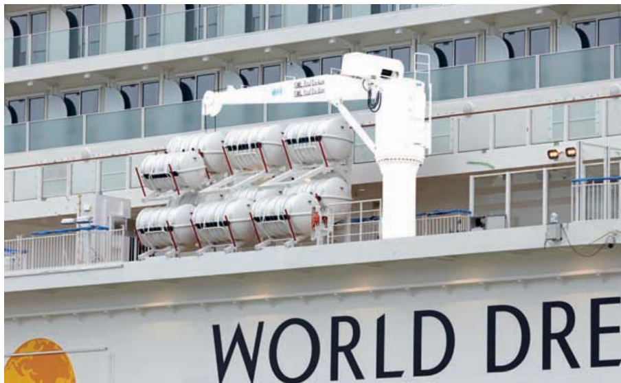
Service crane for liferafts
